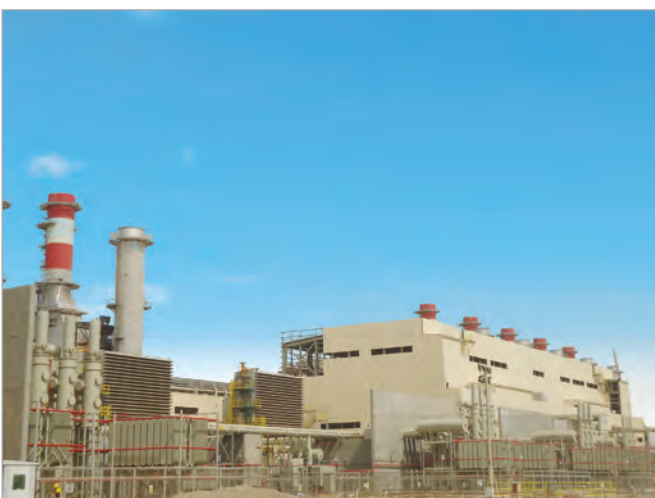
Shoiba Power Plant (KSA)
