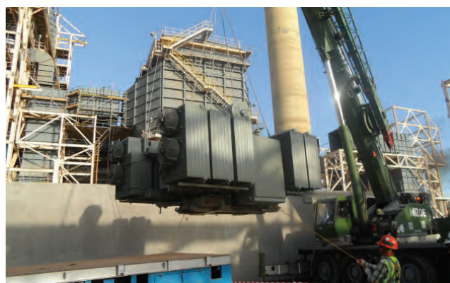
Transformer Rigging
