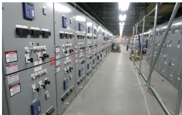
Installation of HVMV SWGR
