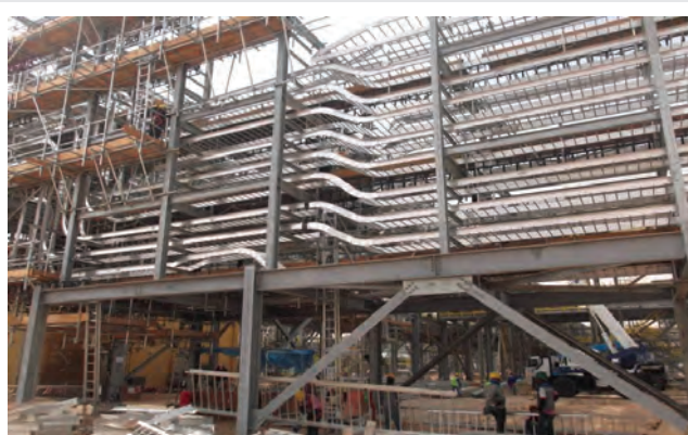
Cable Tray Installation
