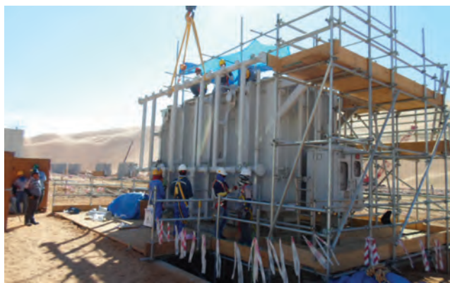
Assembling of Transformer 80MVA
