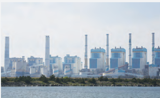
Taeon Thermal Power Plant
