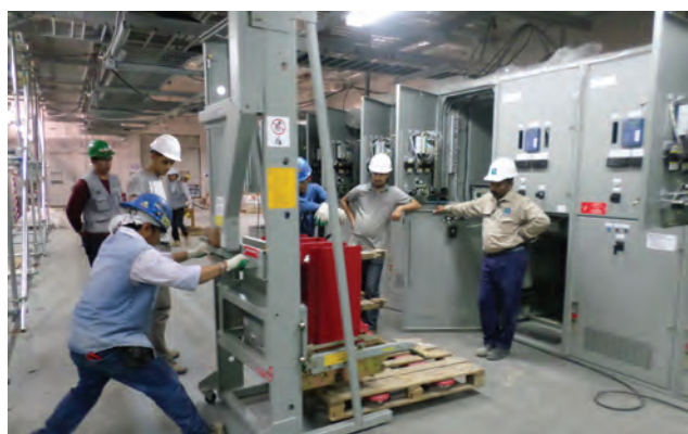
Installation of HV SWGR
