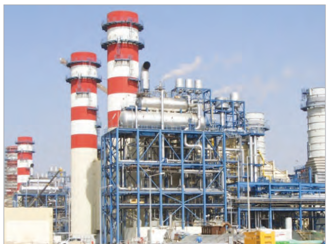
Biskra power Plant [ALGERIA]
