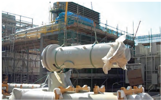
Isolated Phase Busduct(IPB) 3PH 10,000A, 5000A
