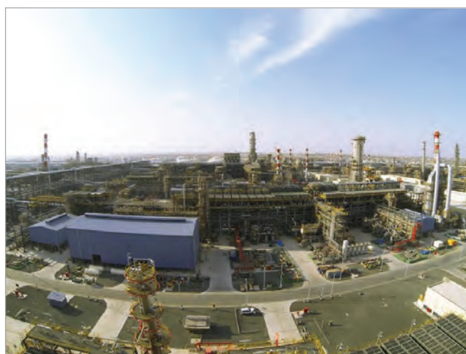
Ruwais Refinery Expansion Project ( UAE )
