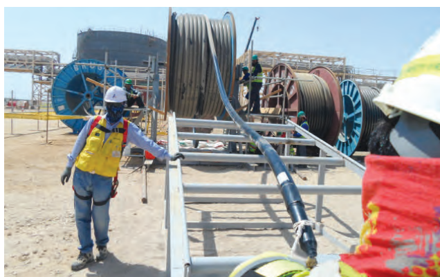
EHV Power Cable Pulling 138KV
