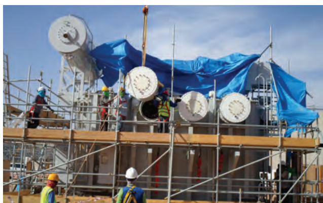
Assembling of Transformer 80-120MVA
