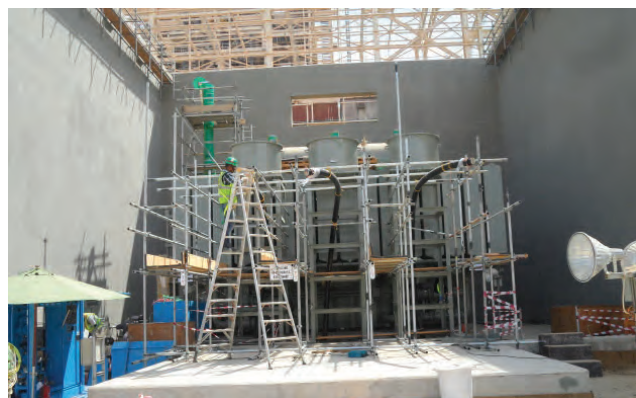
380kV Transformer Erection
