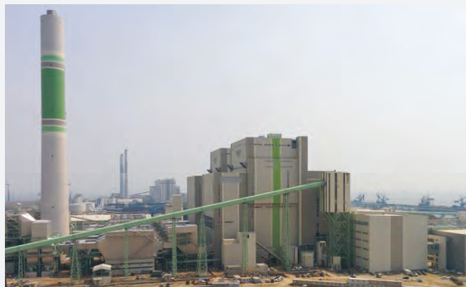
Youngheung Thermal Power Plant
