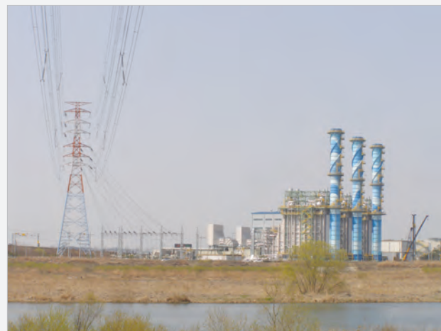
Oh-sung Transmission Line
