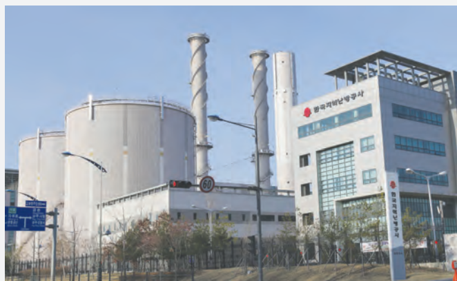
Combined Heat and Power Plant
