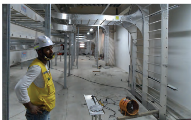
Cable Tray Works
